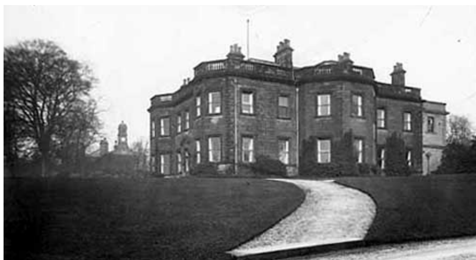
Elmete Hall - View from South West.
